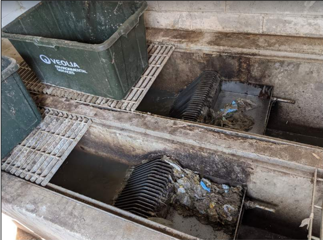
Figure 2. Coarse Screen
