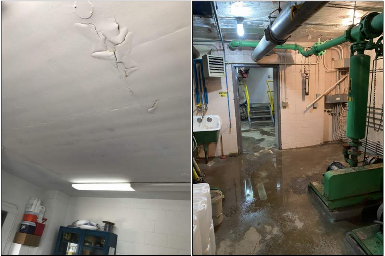
Figure 9. Ceiling and Lower Level of the Main Control Building
